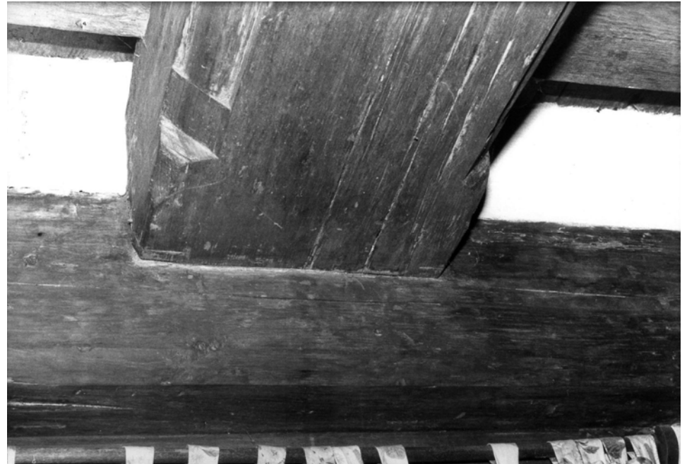
Detail, summer tie beam at south wall, right-hand chamber
