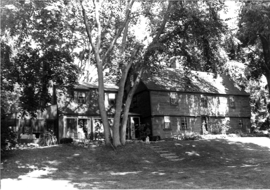
South and west facades
