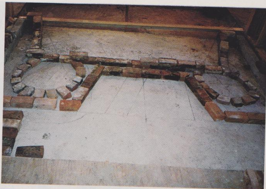
To create a replica of an early chimney, a configuration of back-to-back cooking and parlor fireplaces is laid out in brick. The circular bake ovens will both open from the cooking fireplace.
