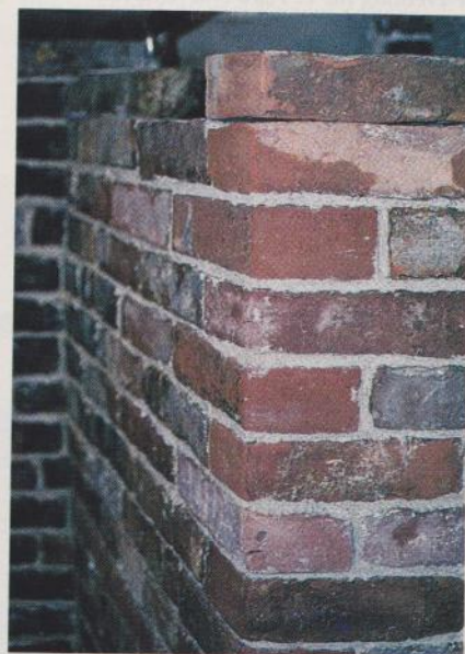
A fireplace under construction replicates an early corner: one clean angle between the front face and the side wall, another between the side and rear walls.
