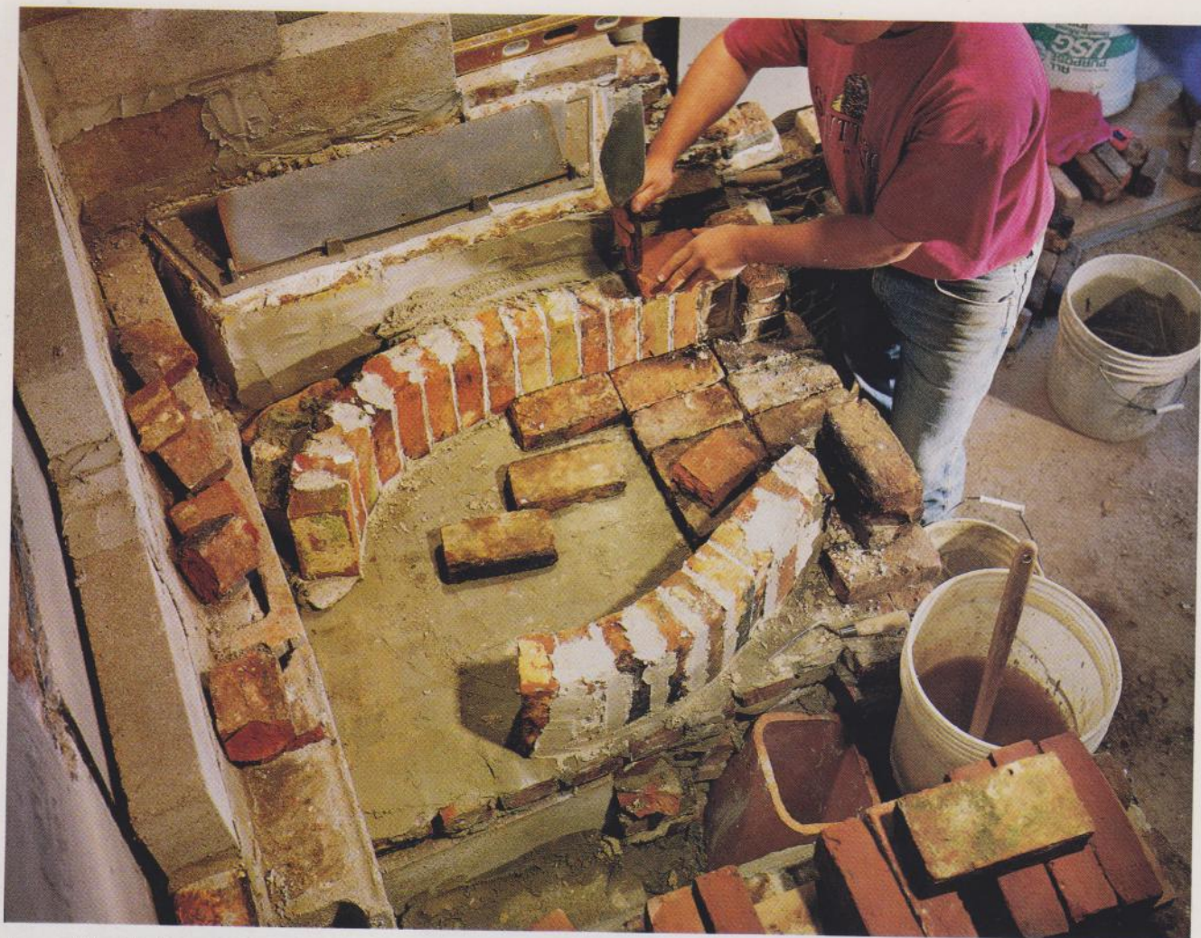
A row of "soldier," or standing, c. 1780 bricks are the starter course for a bake oven in the construction of a new central chimney to replace one removed from a c. 1740 house in Gloucester, Massachusetts.
