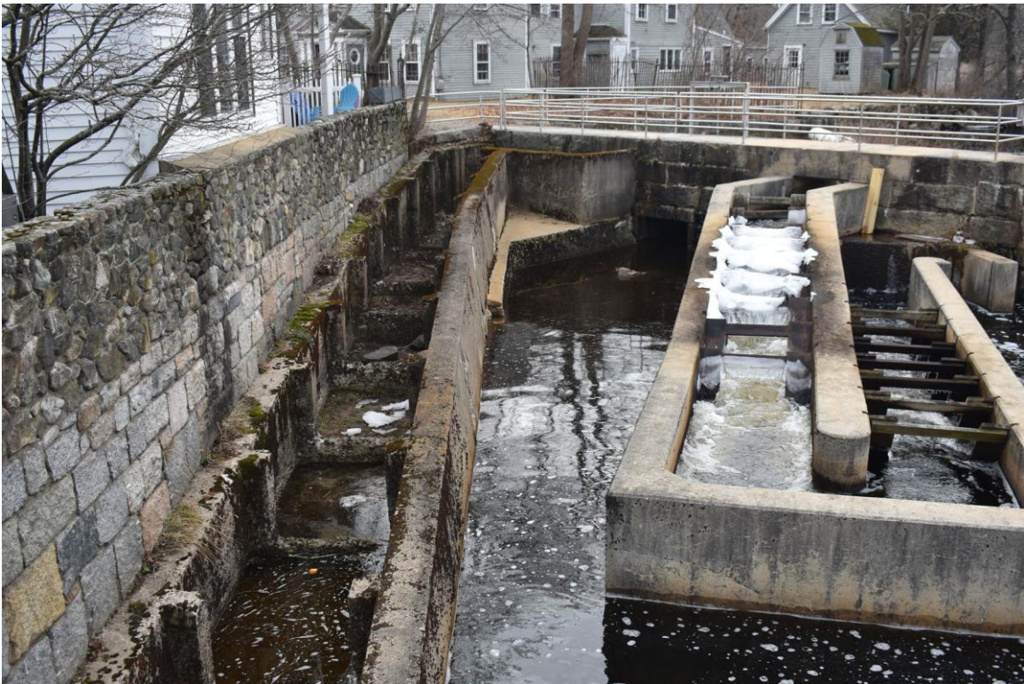
Photo 2. Showing the abandoned (1921) and active Ipswich Mills Dam fish ladders, view south.
