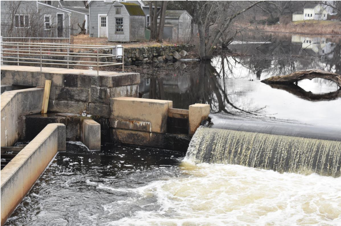
Photo 3. Showing the granite block and concrete masonry of the Ipswich Mills Dam, view south.
